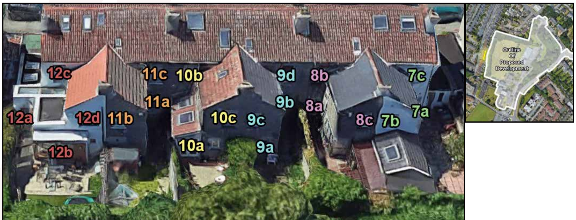
Figure 5.39: Left & Centre - Highlighted areas indicate the position of assessed windows., Right - Aerial view of assessed location
