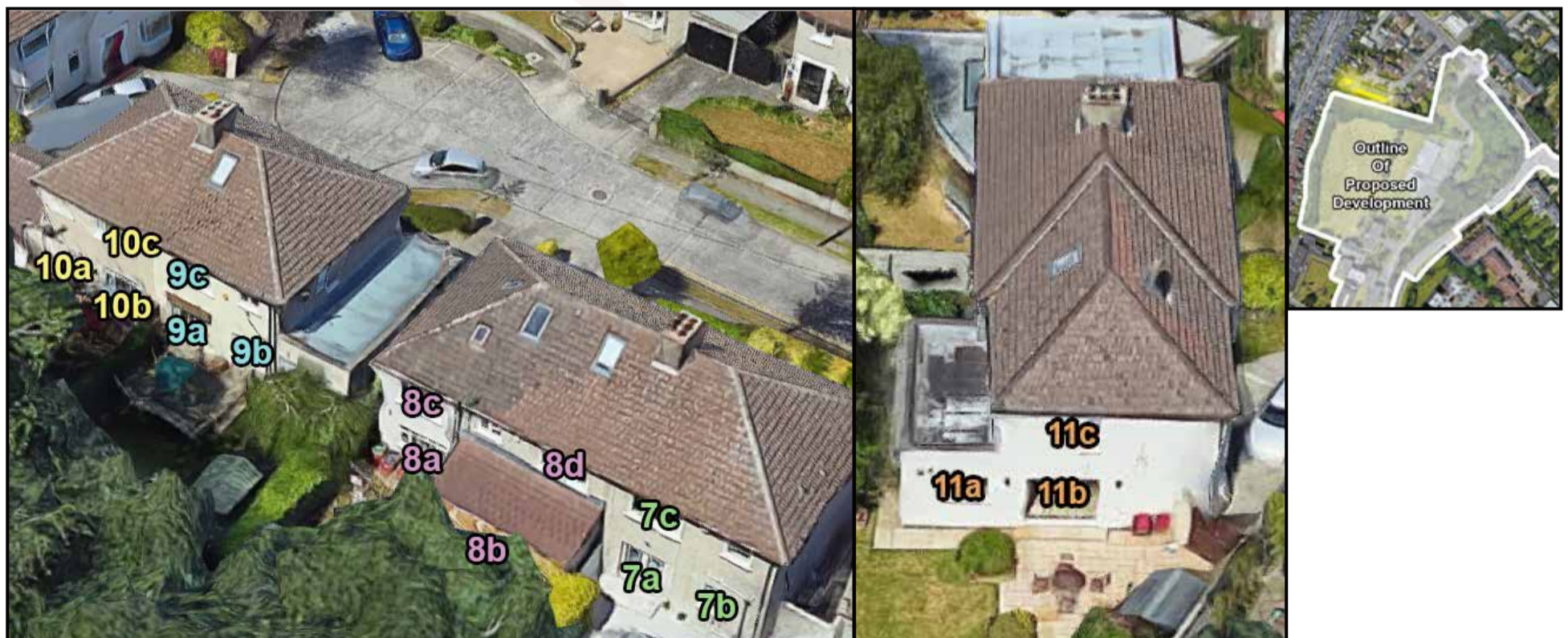
Figure 5.14: Left & Centre - Highlighted areas indicate the position of assessed windows., Right - Aerial view of assessed location
