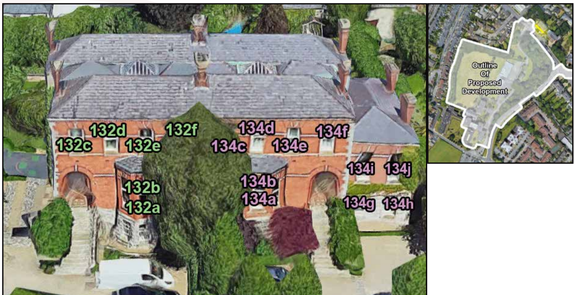
Figure 5.23: Left - Highlighted areas indicate the position of assessed windows., Right - Aerial view of assessed location
