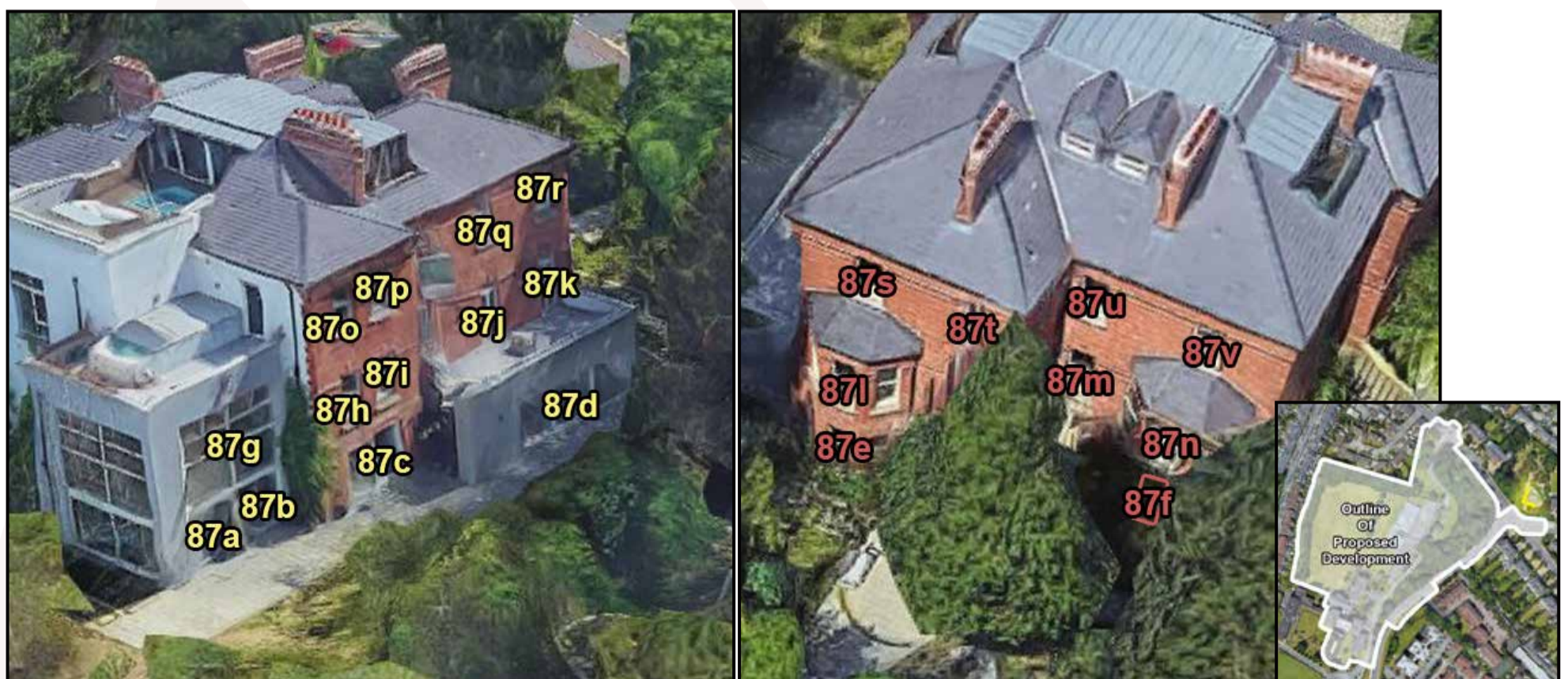
Figure 5.22: Left & Centre - Highlighted areas indicate the position of assessed windows., Right - Aerial view of assessed location
