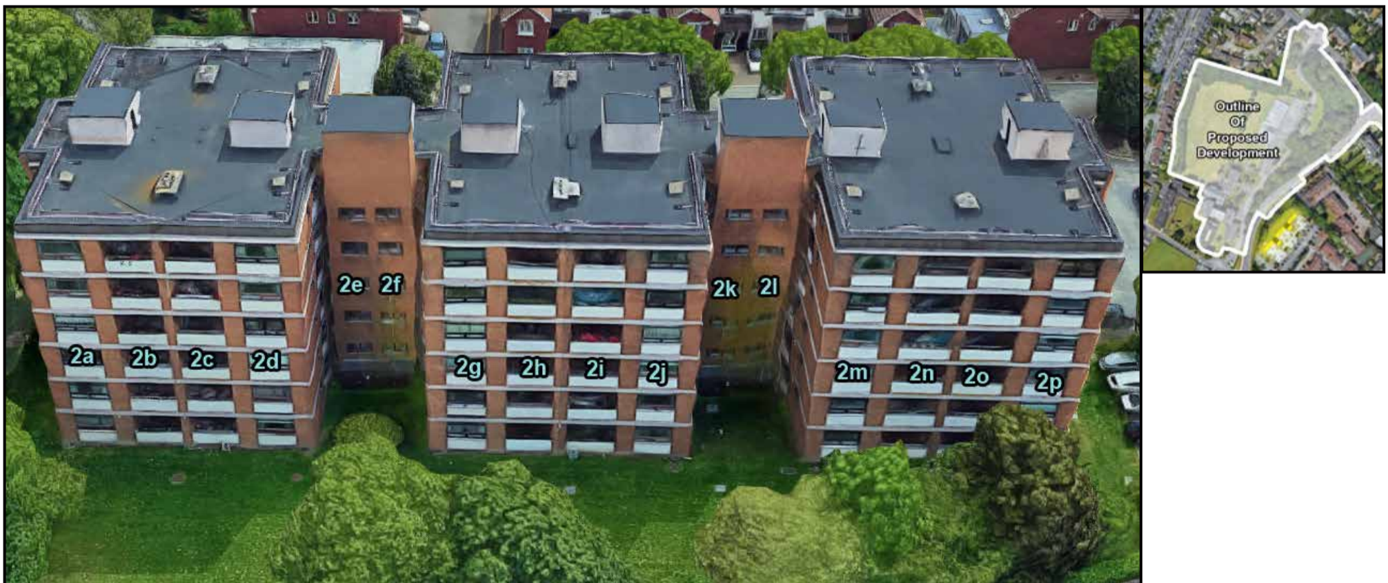
Figure 5.3: Left - Highlighted areas indicate the position of assessed windows., Right - Aerial view of assessed location
