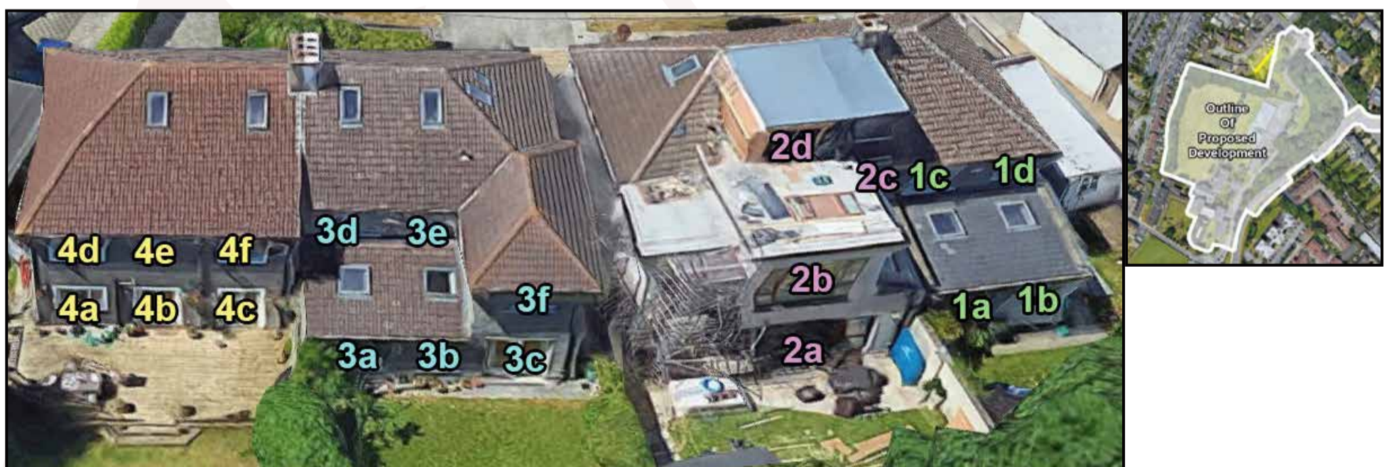
Figure 5.28: Left - Highlighted areas indicate the position of assessed windows., Right - Aerial view of assessed location
