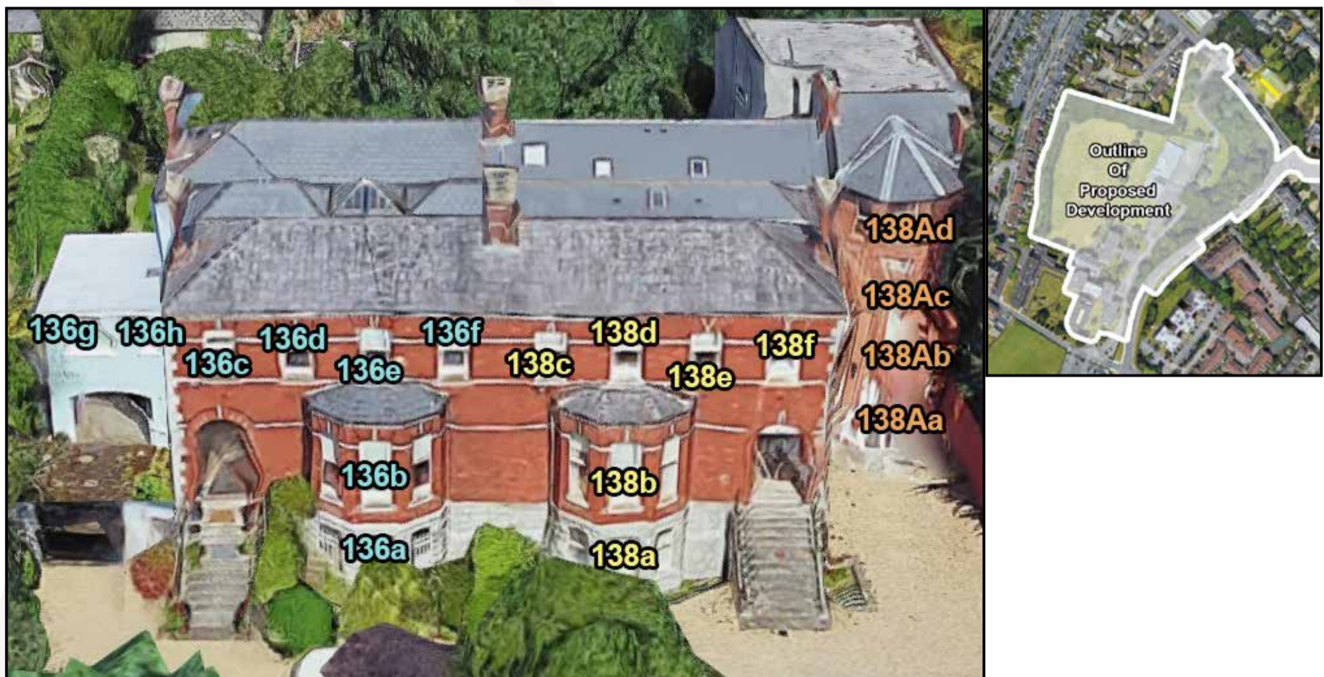
Figure 5.26: Left - Highlighted areas indicate the position of assessed windows., Right - Aerial view of assessed location
