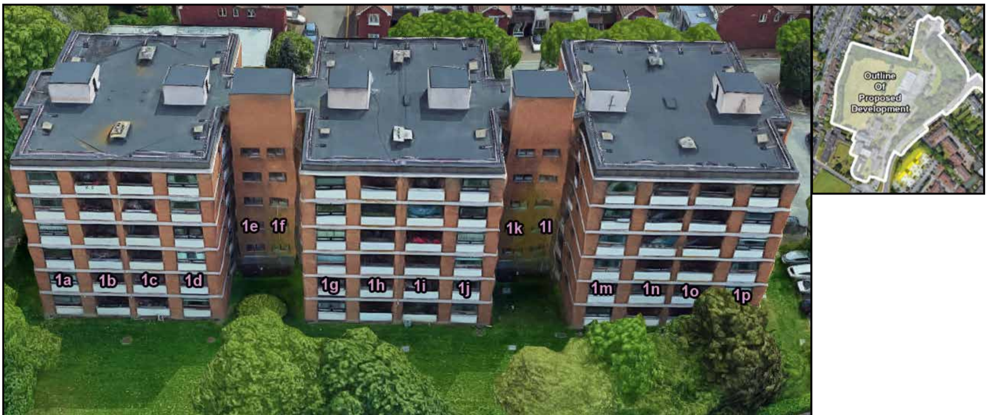
Figure 5.2: Left - Highlighted areas indicate the position of assessed windows., Right - Aerial view of assessed location
