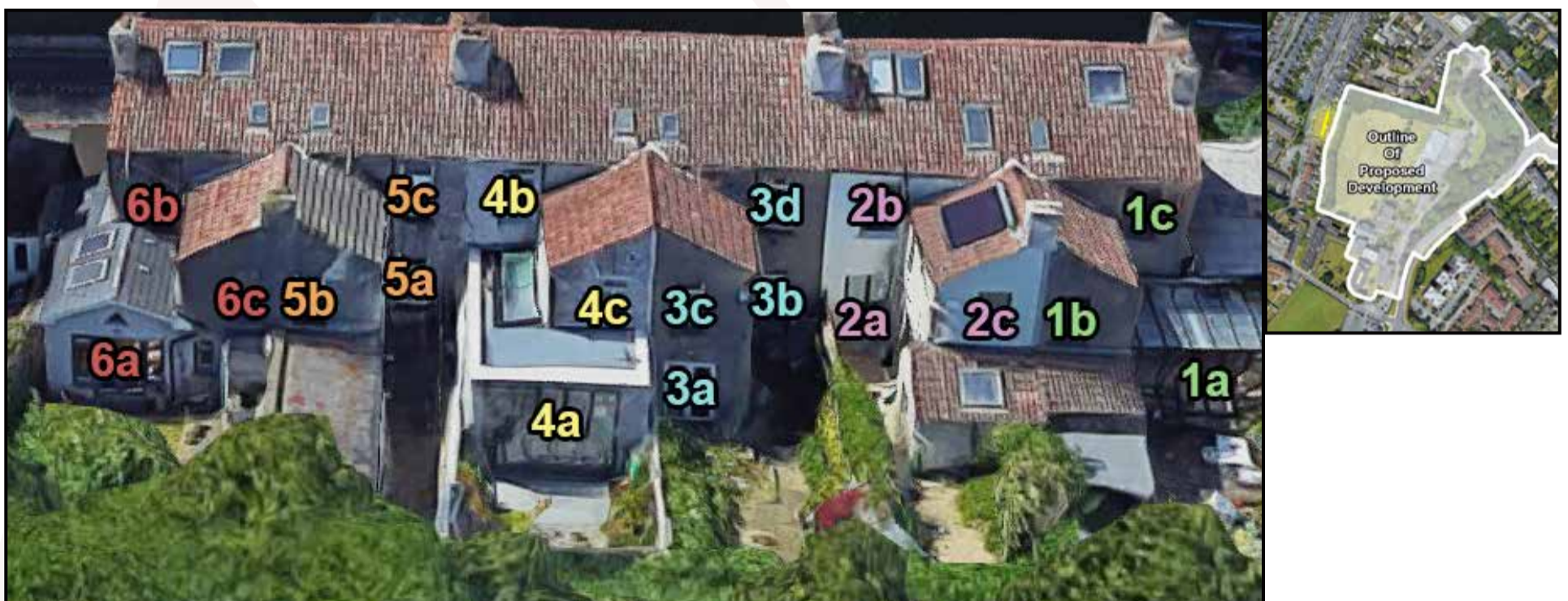
Figure 5.17: Left & Centre - Highlighted areas indicate the position of assessed windows., Right - Aerial view of assessed location
