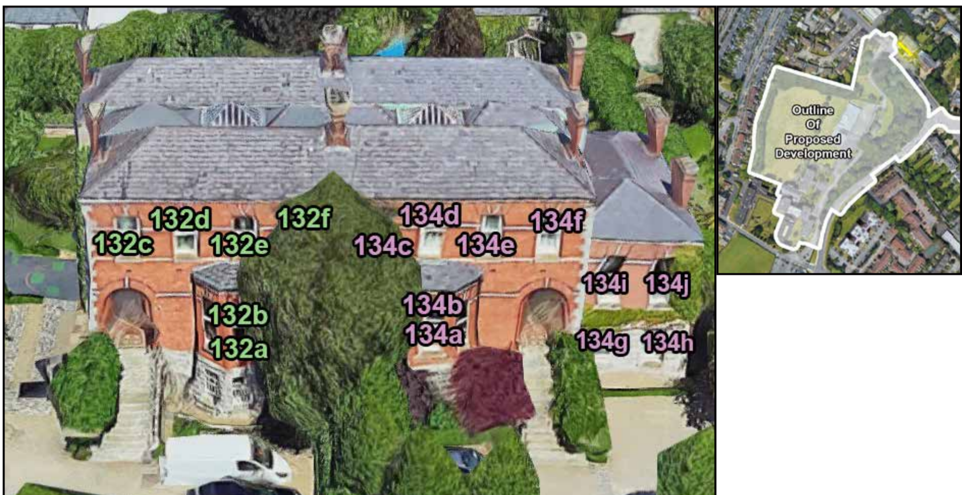
Figure 5.10: Left - Highlighted areas indicate the position of assessed windows., Right - Aerial view of assessed location
