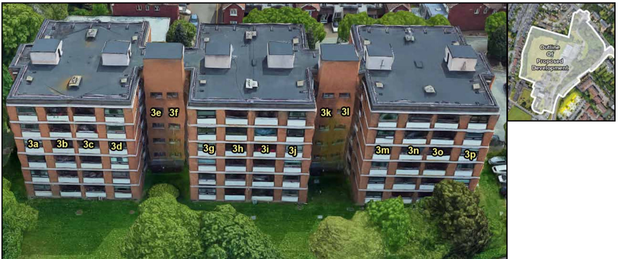
Figure 5.4: Left - Highlighted areas indicate the position of assessed windows., Right - Aerial view of assessed location
