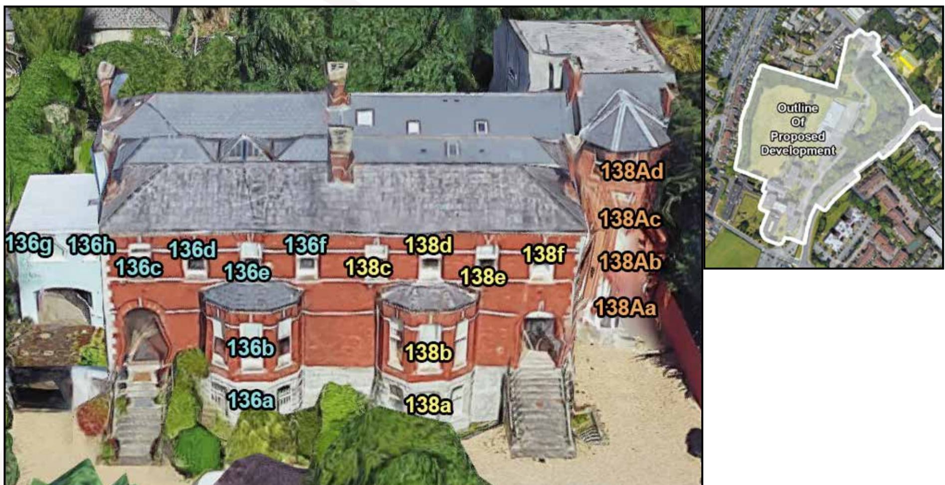
Figure 5.11: Left - Highlighted areas indicate the position of assessed windows., Right - Aerial view of assessed location
