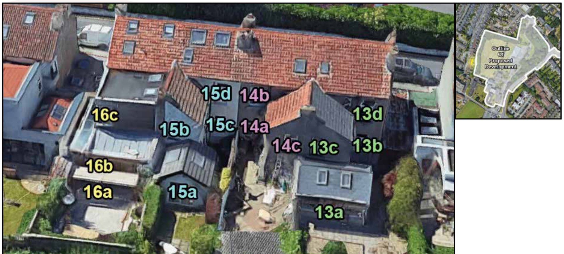
Figure 5.19: Left & Centre - Highlighted areas indicate the position of assessed windows., Right - Aerial view of assessed location
