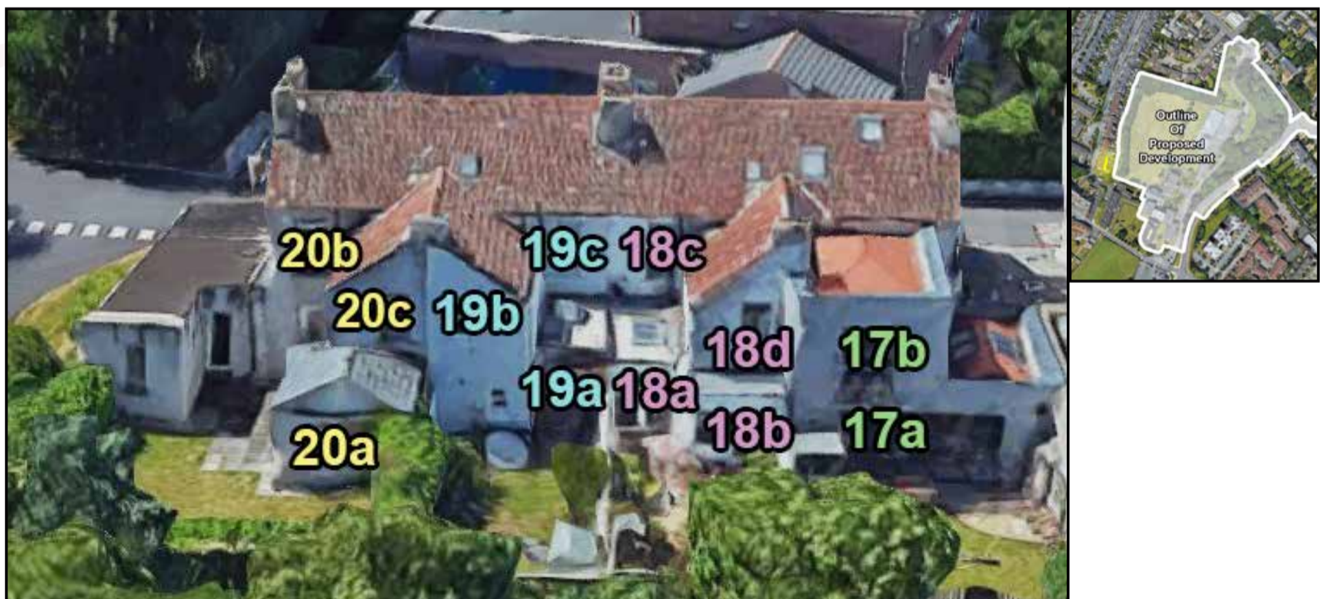
Figure 5.43: Left & Centre - Highlighted areas indicate the position of assessed windows., Right - Aerial view of assessed location
