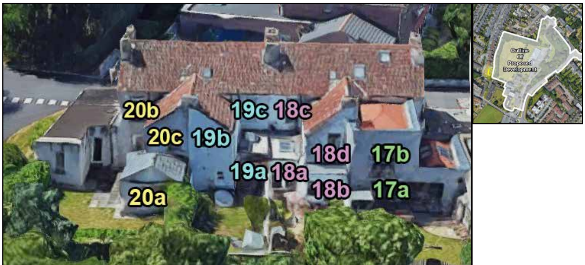
Figure 5.20: Left & Centre - Highlighted areas indicate the position of assessed windows., Right - Aerial view of assessed location
