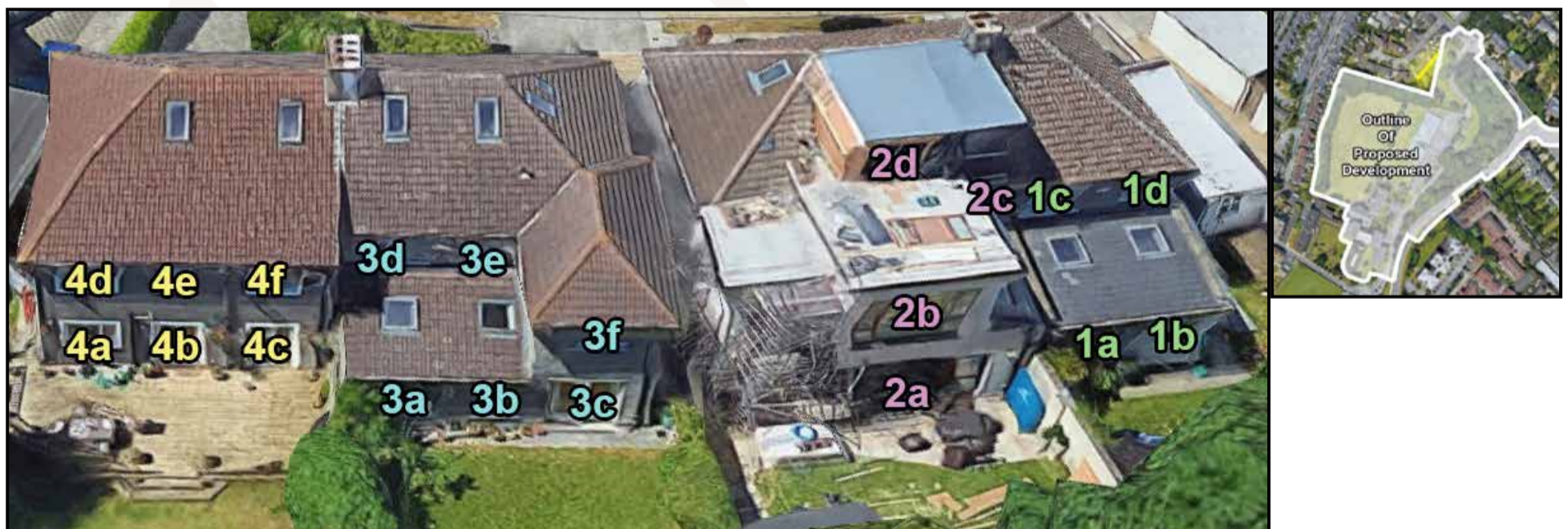
Figure 5.12: Left - Highlighted areas indicate the position of assessed windows., Right - Aerial view of assessed location
