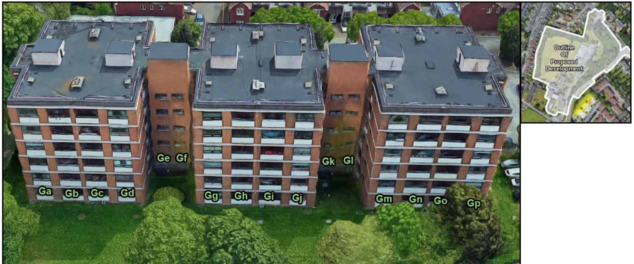
Figure 5.1: Left - Highlighted areas indicate the position of assessed windows., Right - Aerial view of assessed location
