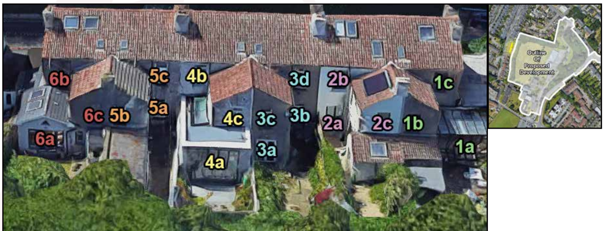
Figure 5.37: Left & Centre - Highlighted areas indicate the position of assessed windows., Right - Aerial view of assessed location
