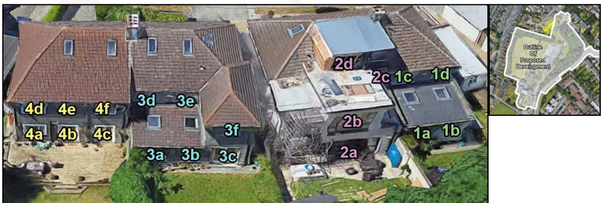
Figure 5.27: Left - Highlighted areas indicate the position of assessed windows., Right - Aerial view of assessed location
