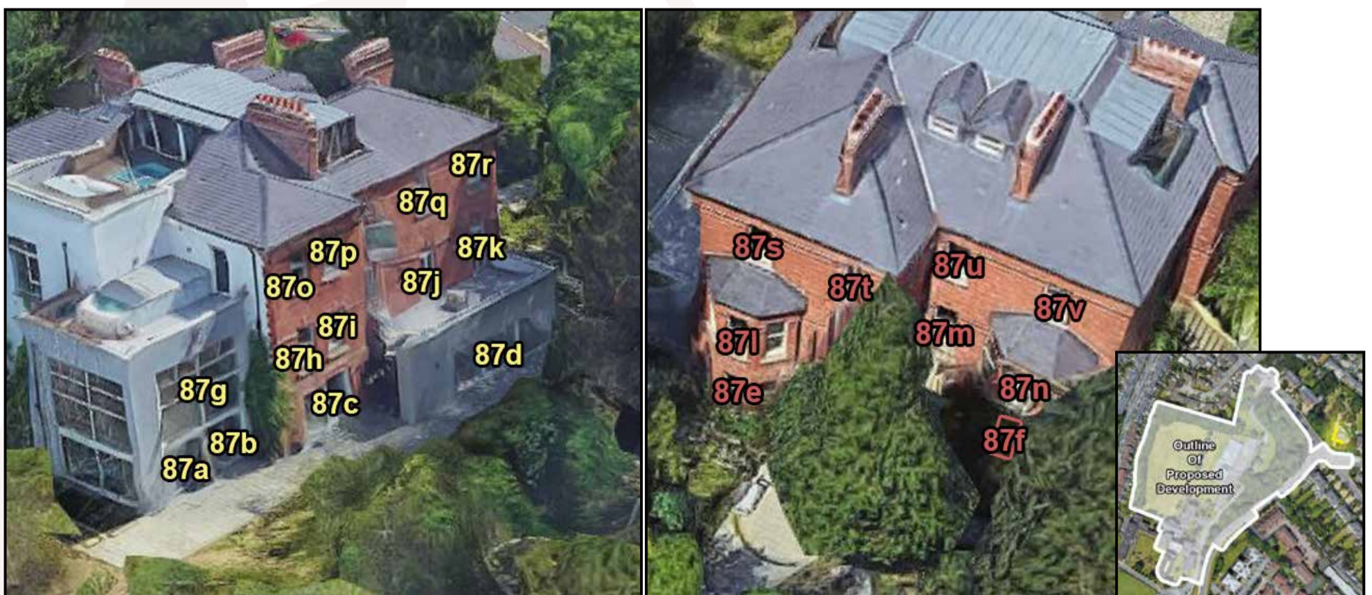
Figure 5.21: Left & Centre - Highlighted areas indicate the position of assessed windows., Right - Aerial view of assessed location
