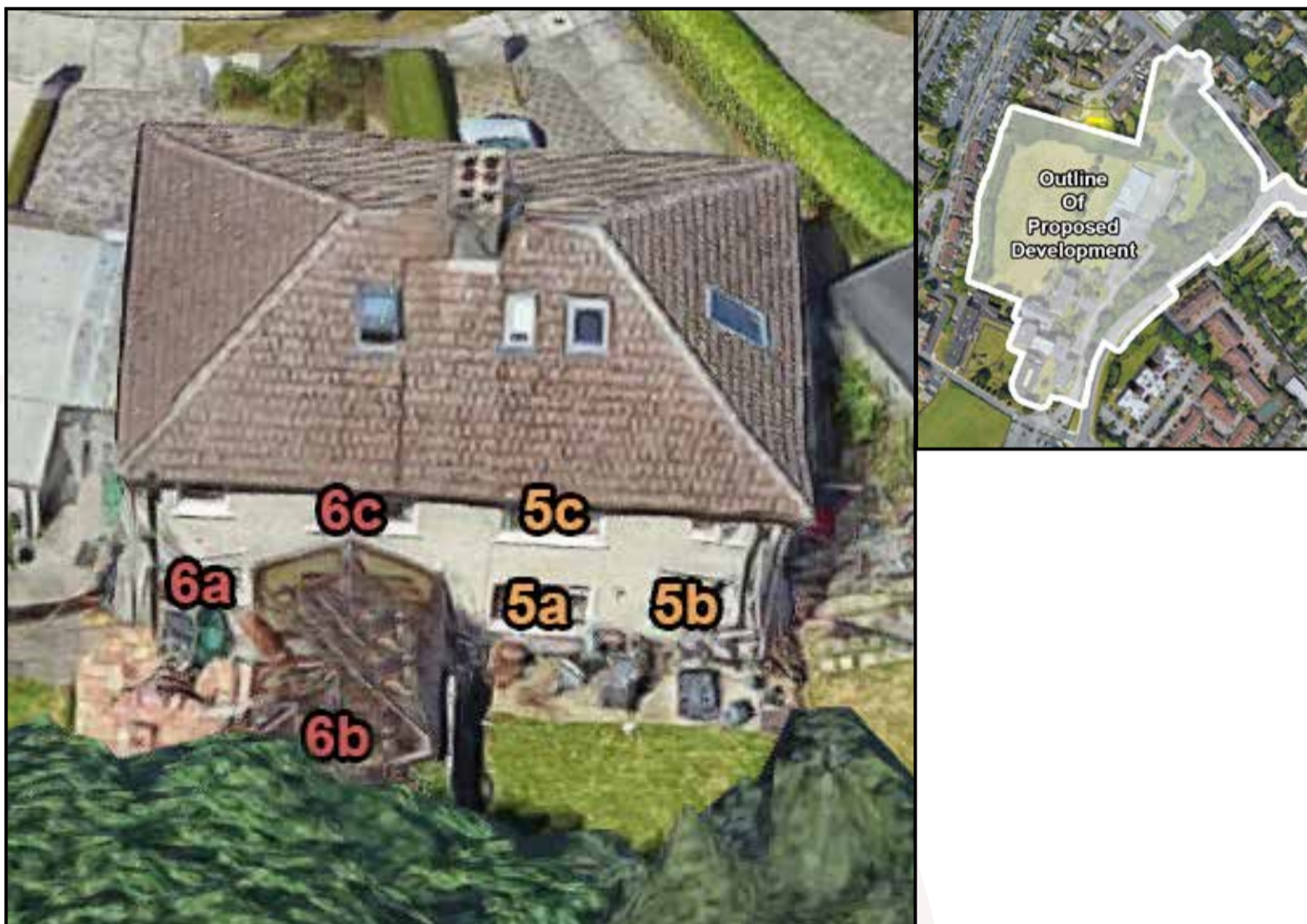
Figure 5.29: Left - Highlighted areas indicate the position of assessed windows., Right - Aerial view of assessed location
