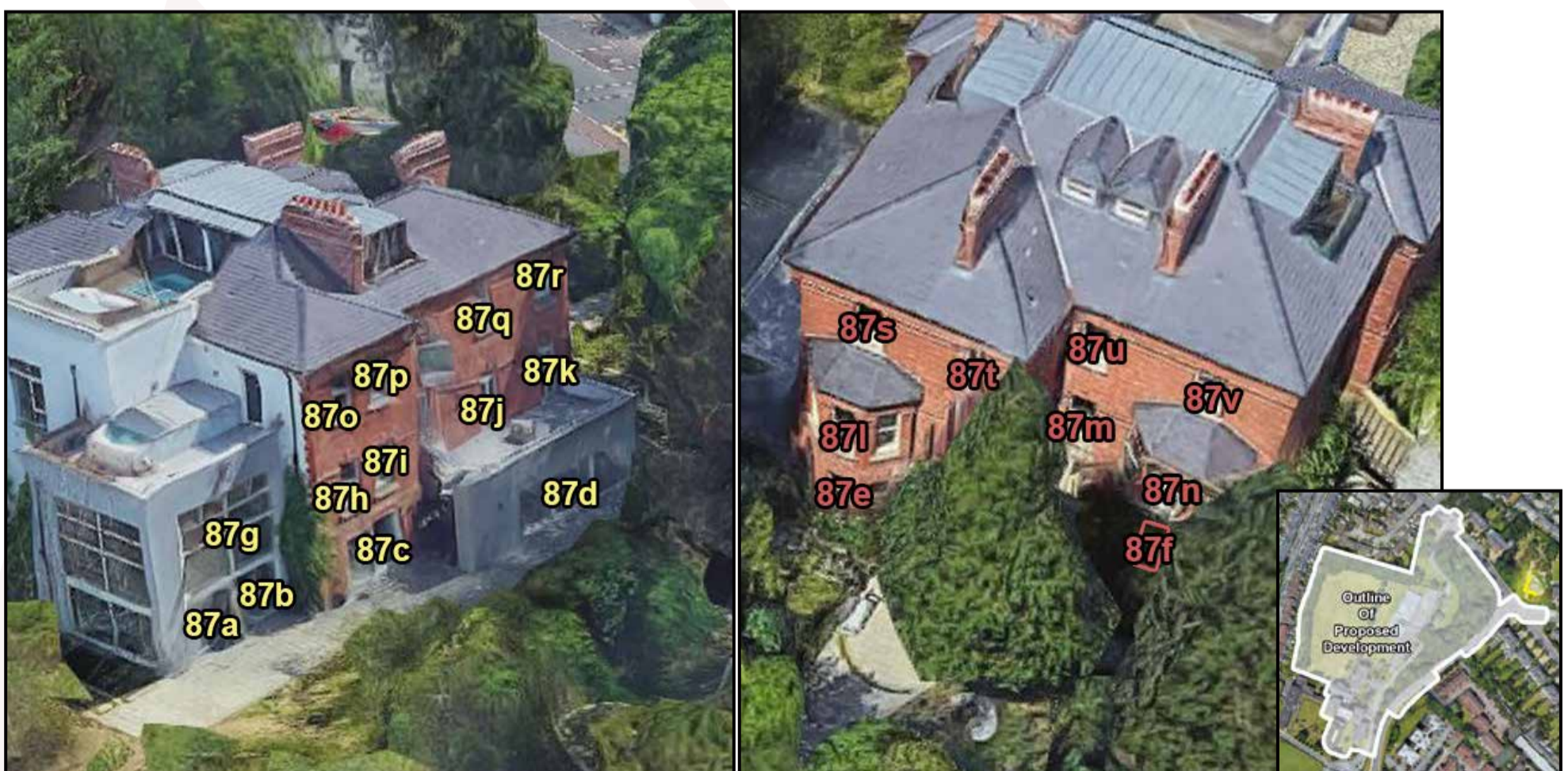
Figure 5.9: Left & Centre - Highlighted areas indicate the position of assessed windows., Right - Aerial view of assessed location
