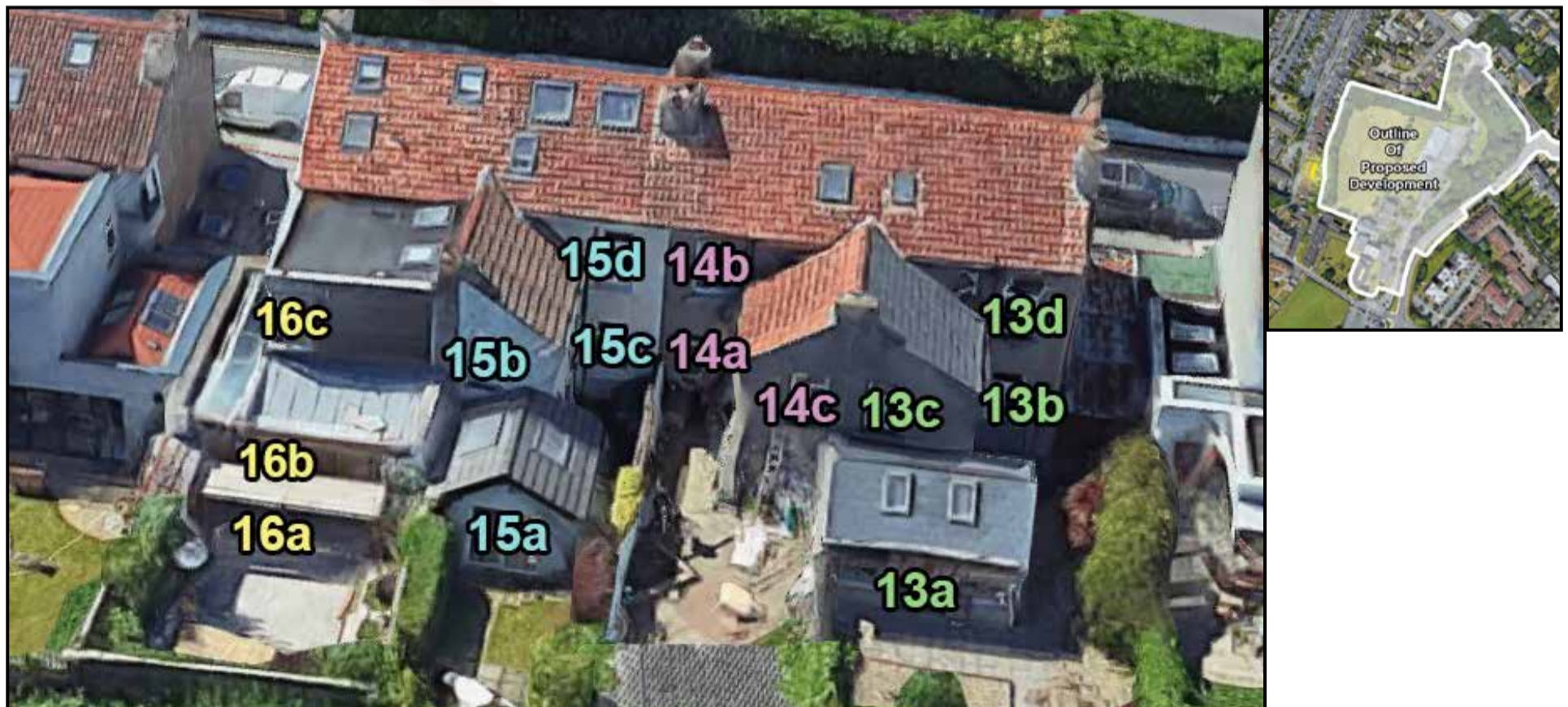
Figure 5.42: Left & Centre - Highlighted areas indicate the position of assessed windows., Right - Aerial view of assessed location
