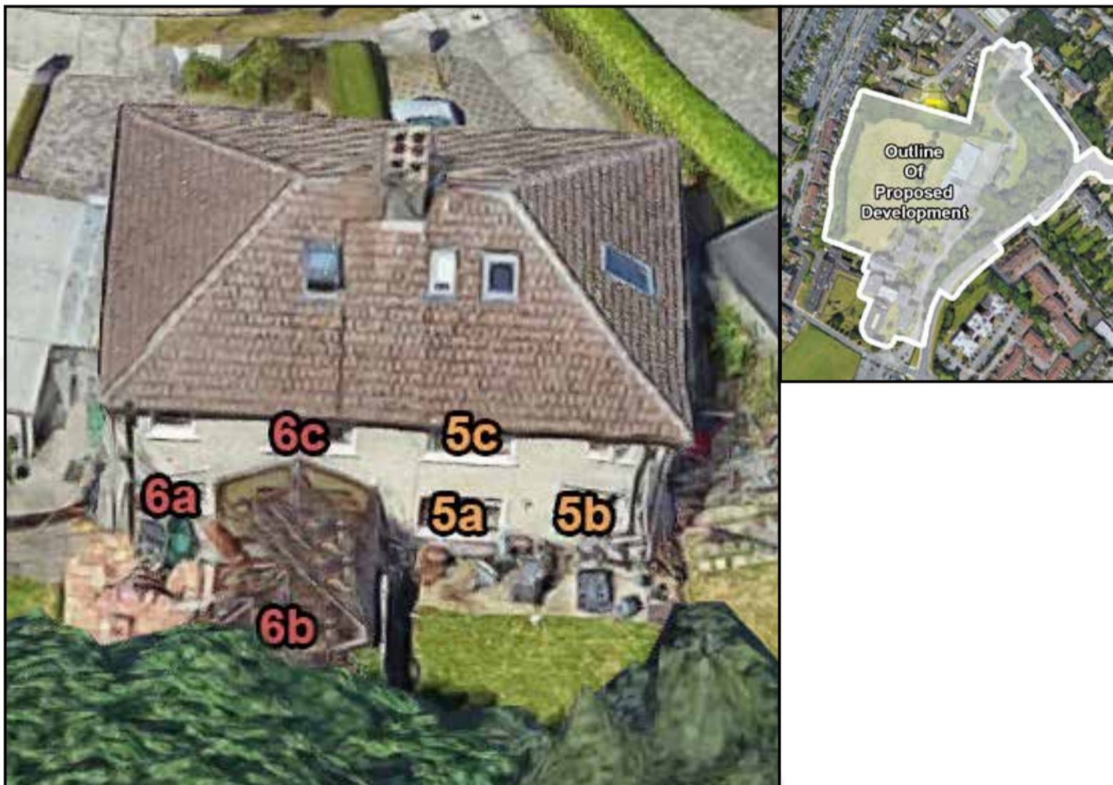
Figure 5.13: Left - Highlighted areas indicate the position of assessed windows., Right - Aerial view of assessed location
