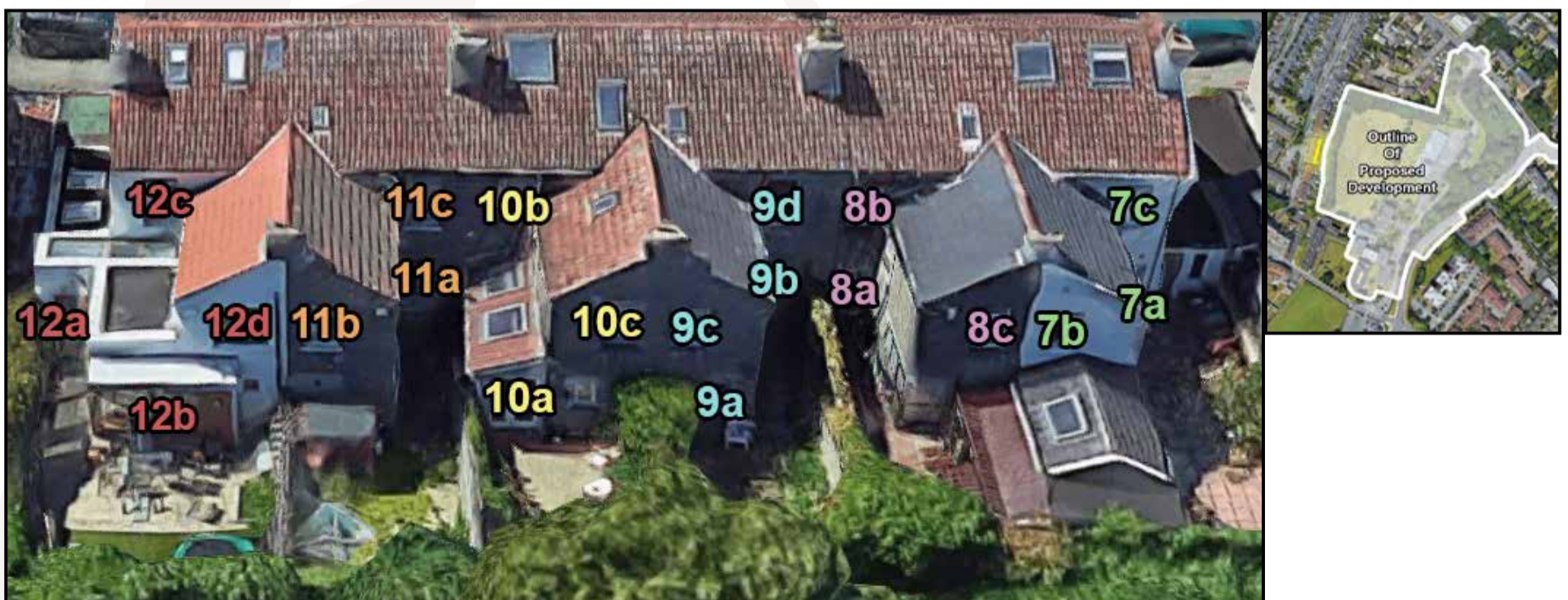
Figure 5.18: Left & Centre - Highlighted areas indicate the position of assessed windows., Right - Aerial view of assessed location
