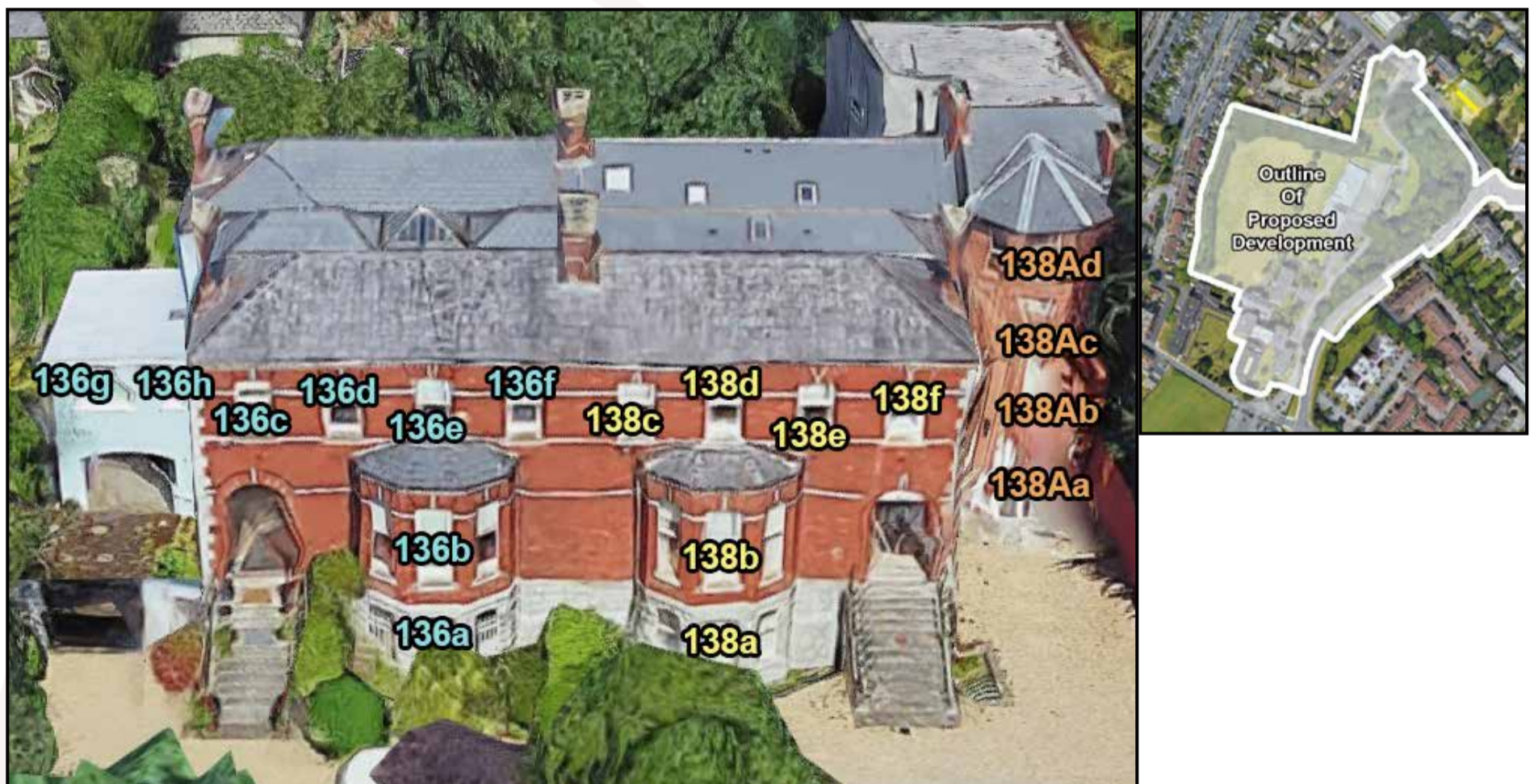
Figure 5.25: Left - Highlighted areas indicate the position of assessed windows., Right - Aerial view of assessed location
